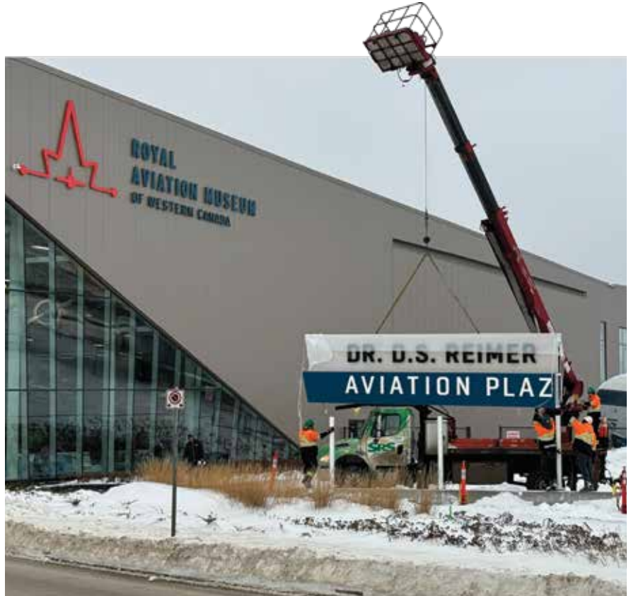
Sign Installation January 24, 2024
